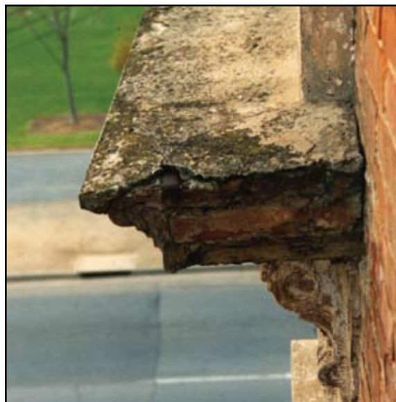
Lack of maintenance on top surface of cornice has allowed water to seep in and damage the moulding.
